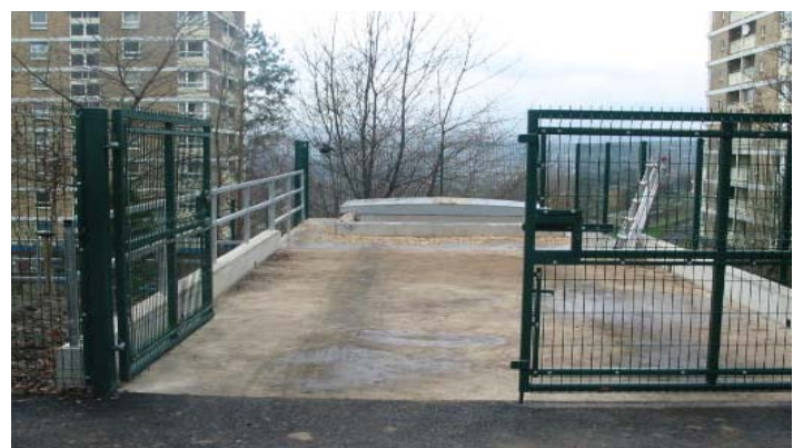
Fuel reception bunker
