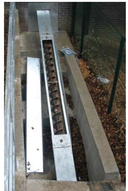
20m auger from fuel reception to internal bunker
