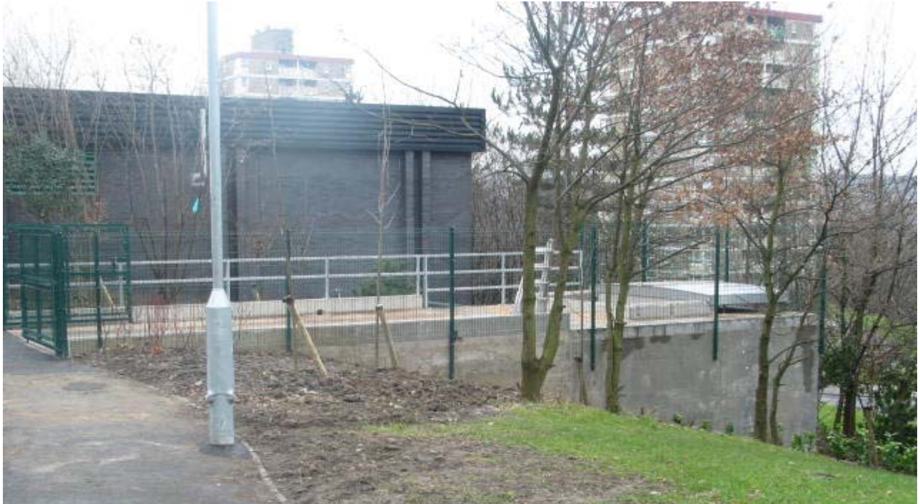
Boiler room (behind) & fuel reception bunker
